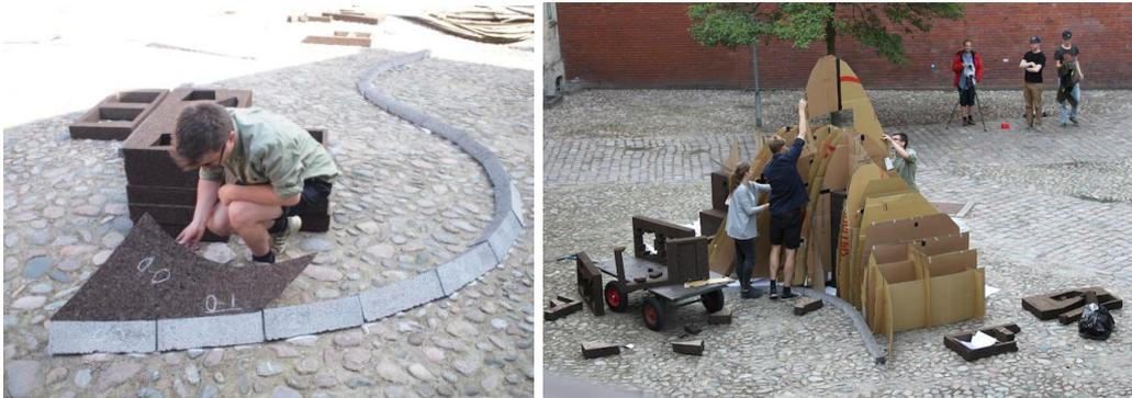
Figure 4: Construction of the vault (Left) Test-fitting the voussoirs. (Right) Constructing the cardboard centering.
